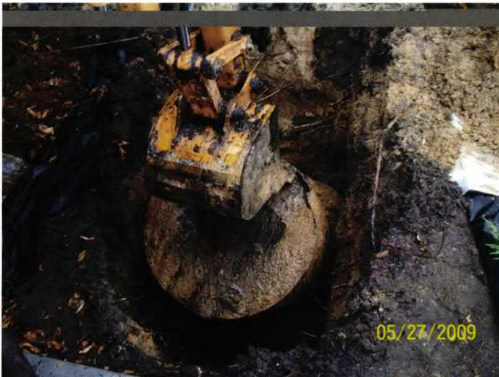
Picture 2: UST 1040Iris during removal.
