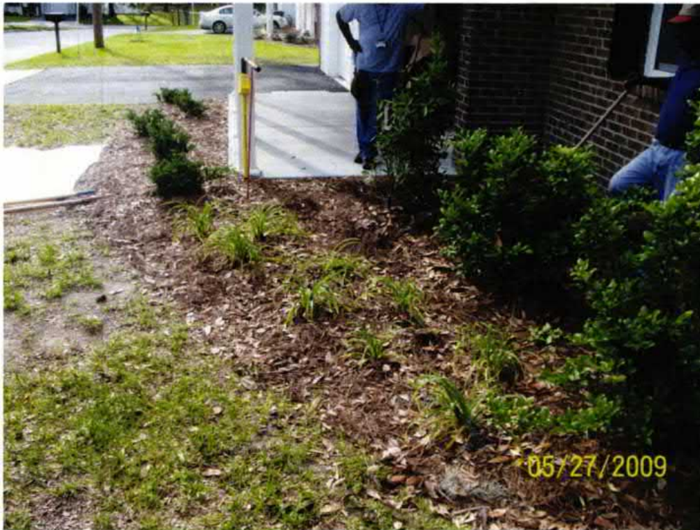
Picture 1: Location of UST 1040Iris prior to excavation.
